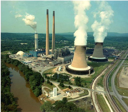
Coal power plant
